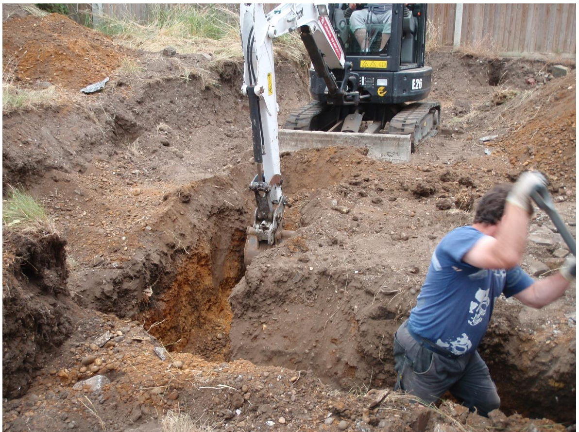
Plate 3 Excavation of the foundation trenches (note the level of ground reduction)
